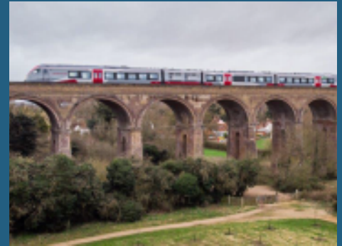
New train over Chappel viaduct
